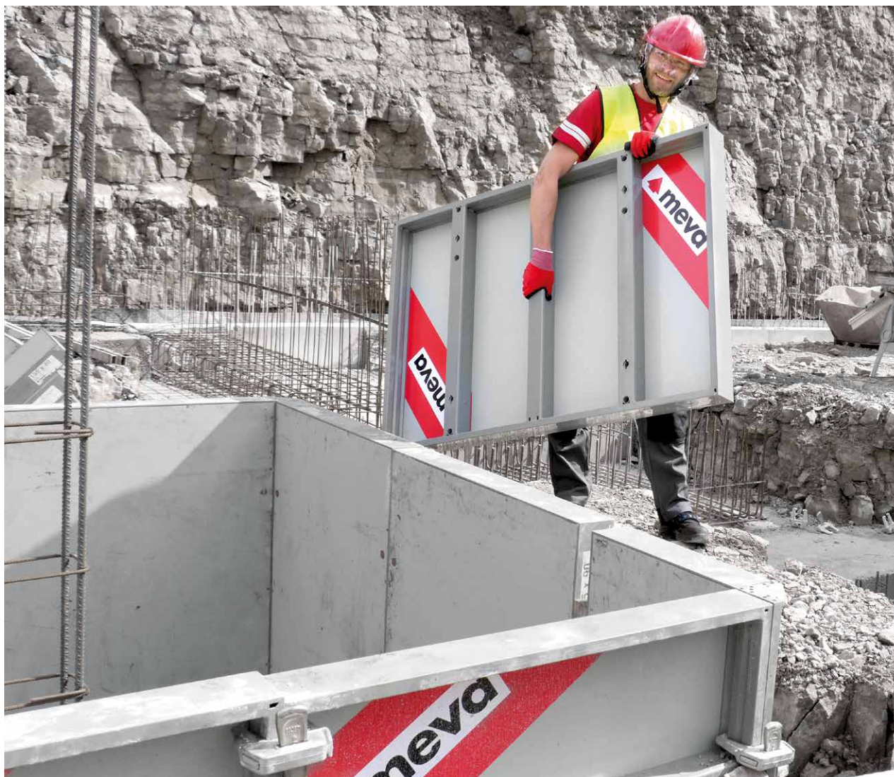
The low panel weight and ergonomic grip profile ensure safe, non-strenuous working.
